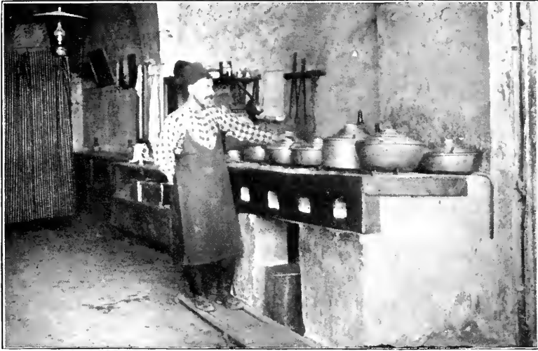
In the Turkish restaurants food is cooked over holes in a limestone slab, while below the charcoal fire is fed through other openings which also make the draught.
